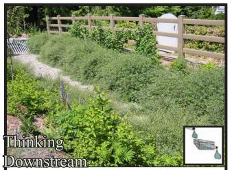
As rain washes over the built landscape, it may be contaminated by oil and grease, heavy metals, pet waste, chemical fertilizers and pesticides. In the 110th St. Cascade design, water quality is improved when polluted sediments settle out in catchbasins. Plants, soils, and natural river rock in the swale further filter out sediments organically as runoff passes through the system. Bacteria in healthy soils can also help break down carbon based pollutants like motor oil.
